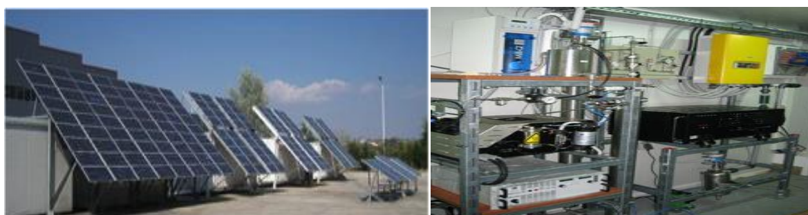
Figure 35. Xanthi. Islanded RES-powered microgrid with battery stacks and hydrogen storage at SUNLIGHT premises
